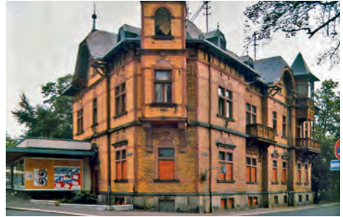
The Ploß-Villa before its demolition
