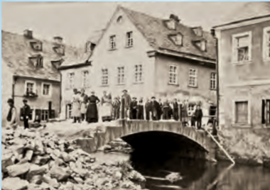
Construction of the Selbbach Bridge on the Hohenberger Straße - approximately 1921
